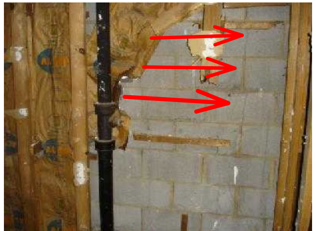
Stress Cracks
