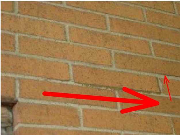
Foundation Cracks
