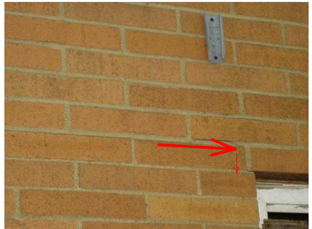
Stress cracks
