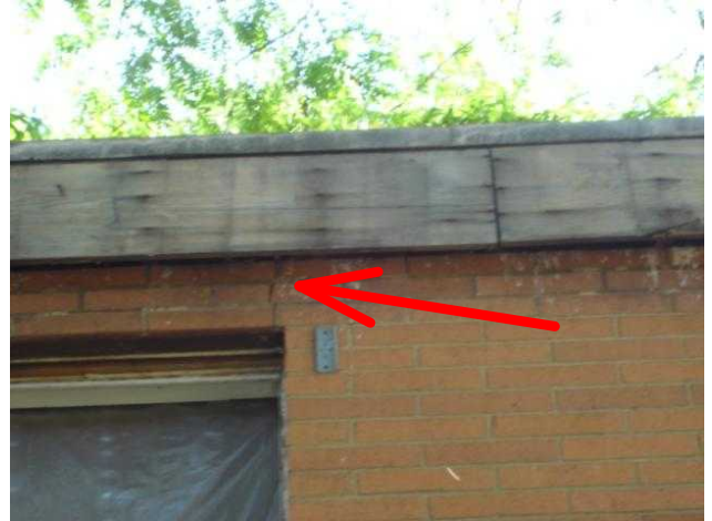
Stress Cracks
