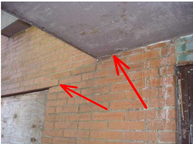
Stress Cracks
