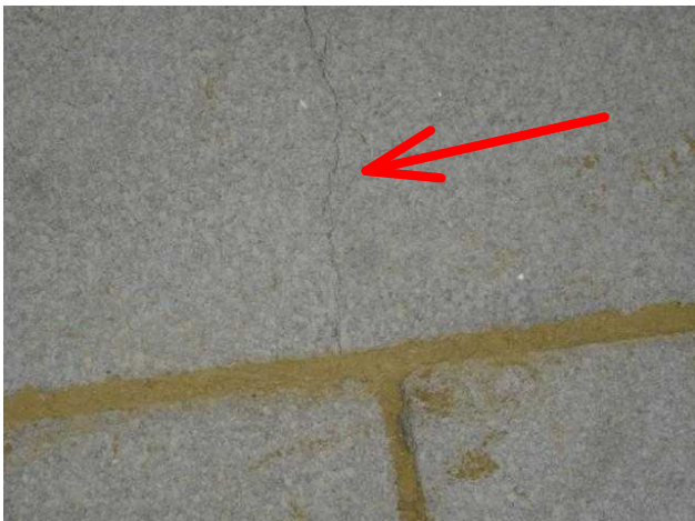
Stress Cracks
