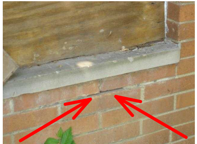
Stress Cracks
