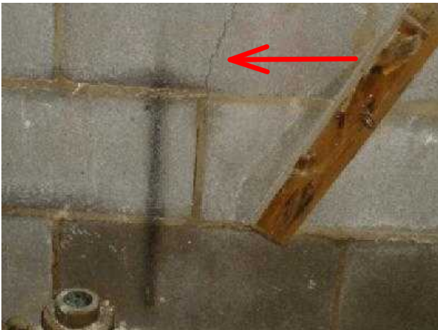
Stress Cracks
