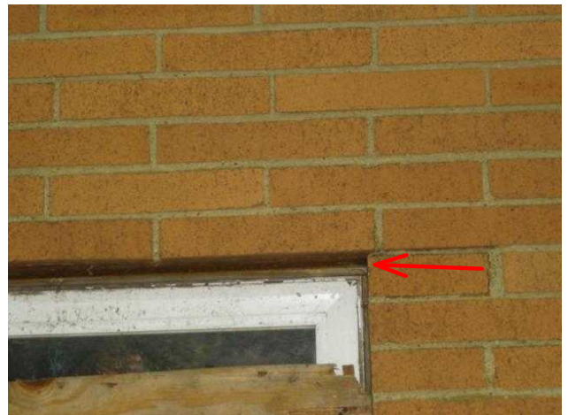
Stress cracks
