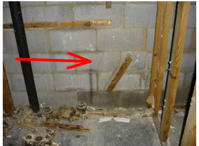
Stress Cracks
