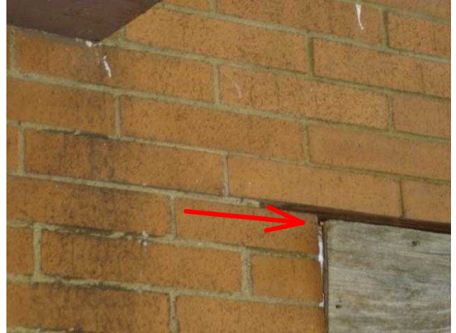
Stress Cracks
