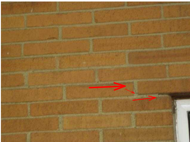
Stress cracks
