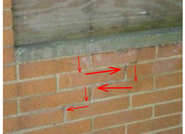
Foundation Cracks
