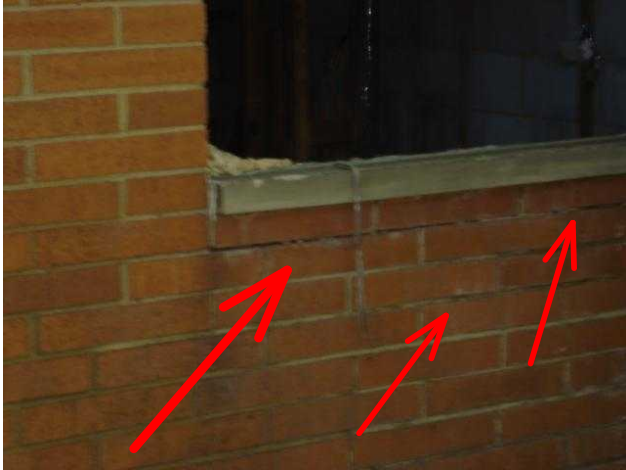
Stress Cracks
